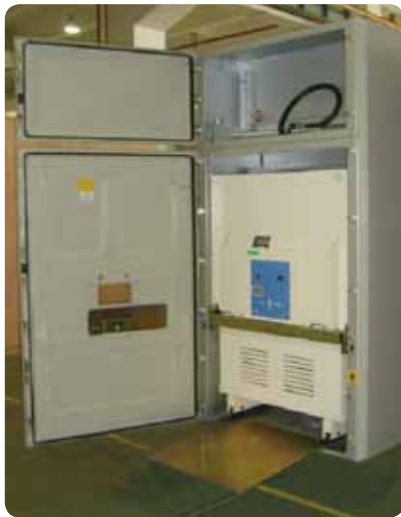
Fig.5.4 The floor rolling circuit breaker access the cubicle
