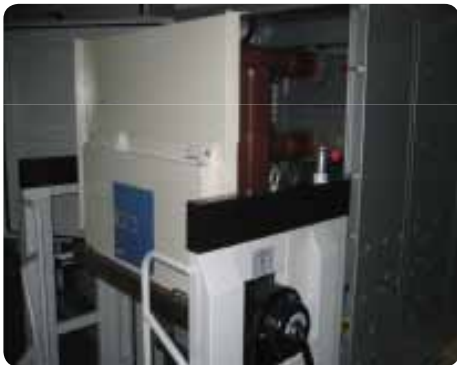
Fig. 5.2 Couple the transport truck to the Panel
